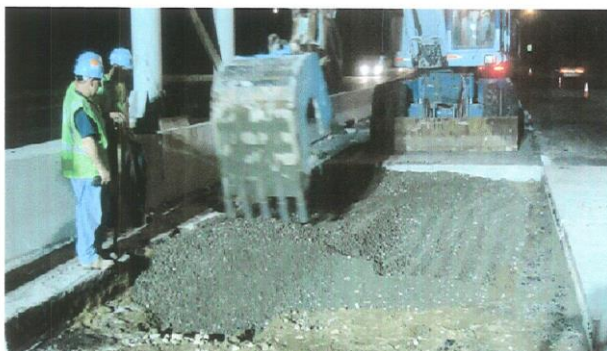
Figure 6. Removal of old pavement.
