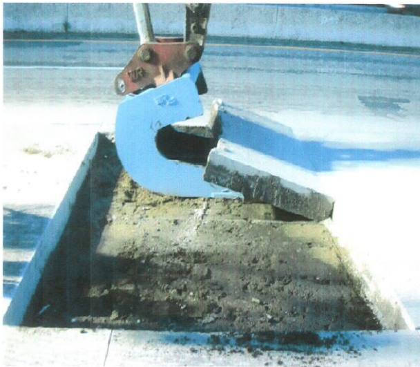
Figure 6. Removal of old pavement.
